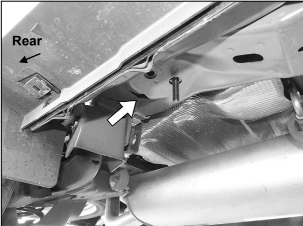
(Fig 20) "Short" Bolt Plate installed (arrow)
